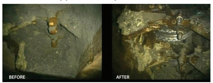
The OC Robotics JetSnake arm is equipped with a high pressure water jet for cleaning and a camera and lights for real time process monitoring and inspection.
